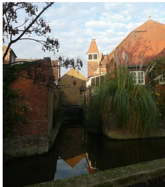
The Cornmill Stream running under the Town Hall (EFDC)
