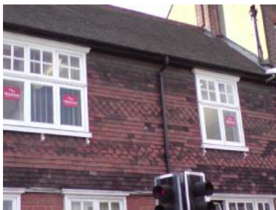
Hanging tiles (EFDC)
