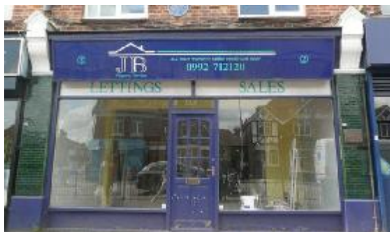
Tiled pilaster with decorative console (EFDC)
