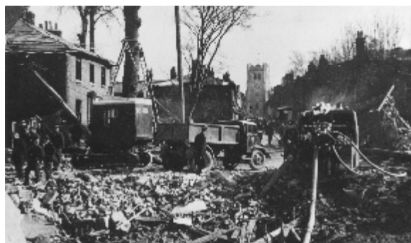
Bomb damage in Highbridge Street (Reflections of the Past, R. Sears & J. Foster)
