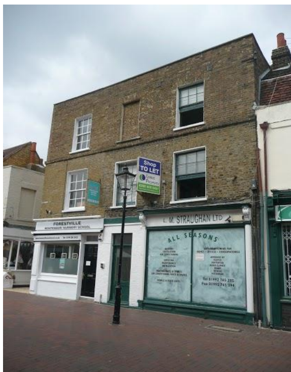
Vacant shops, Sun Street (EFDC)
