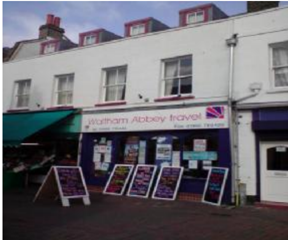
Large adverts and excessive signage (EFDC)
