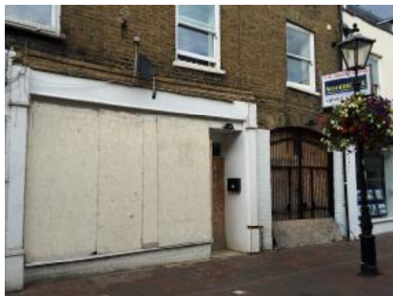
Vacant shops, Sun Street (EFDC)
