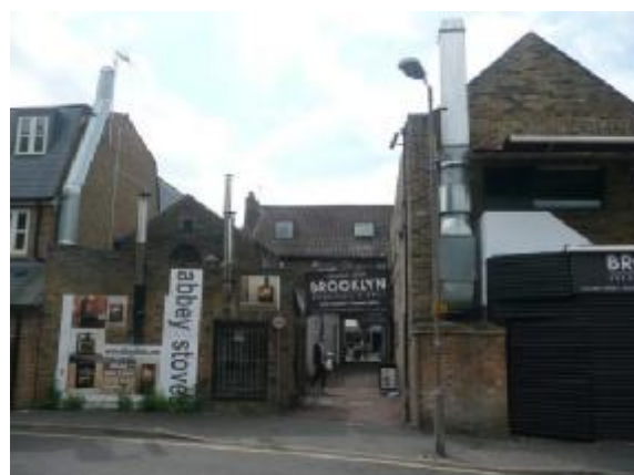
Unsympathetic alterations to buildings, Darby Drive (EFDC)
