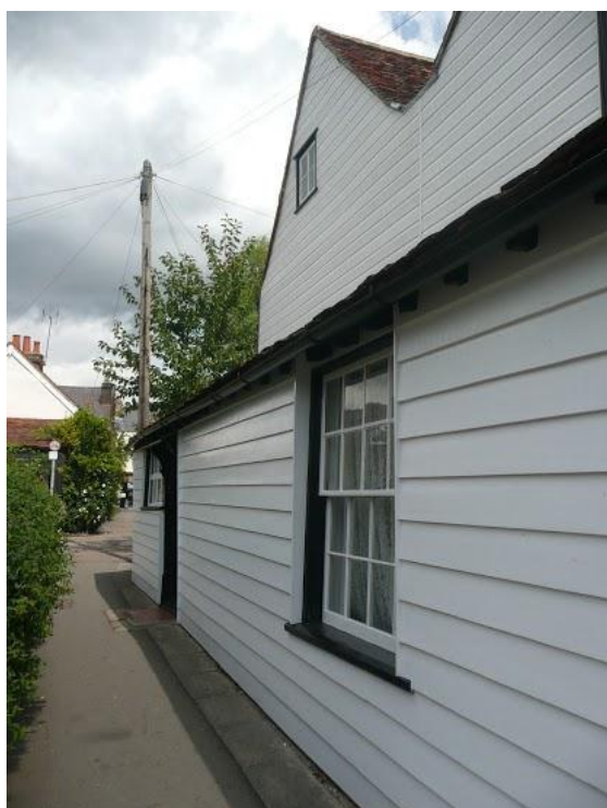
Weatherboarded cottage, South Place (EFDC)
